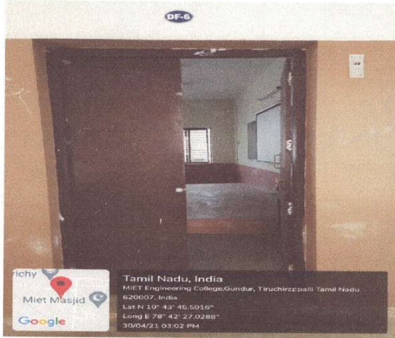
DF6 - Entrance of the Class Room
