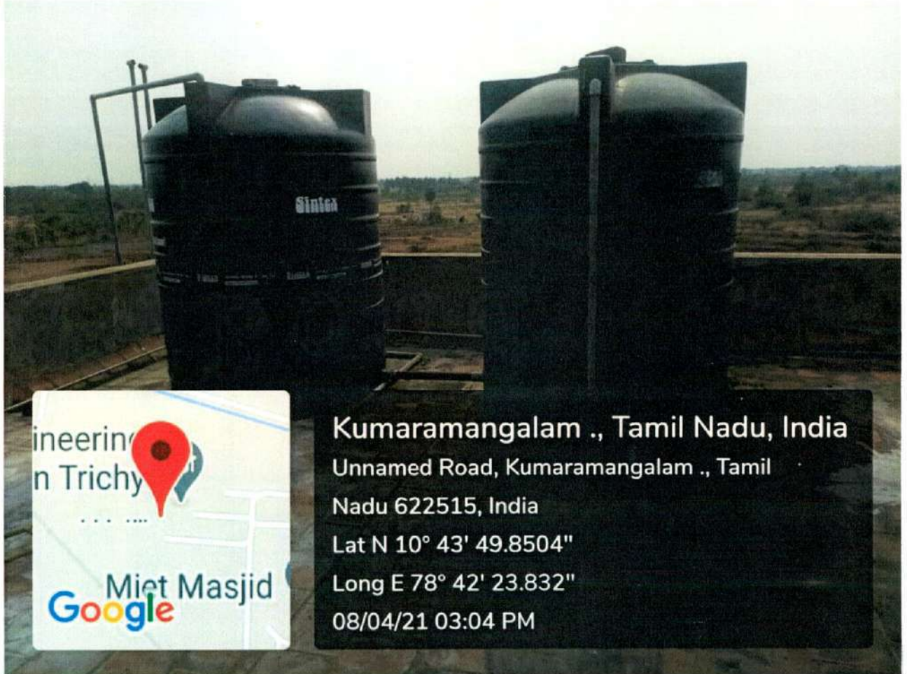
Construction of Water tanks
