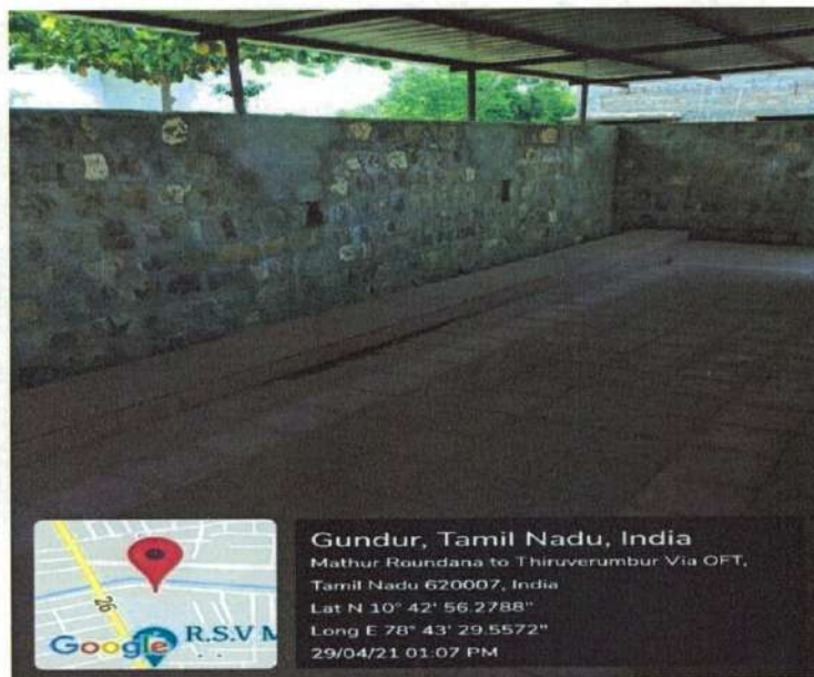
Toilet construction at Government Special Higher Secondary School, Mathur
