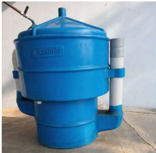
0.5 M 3 Capacity Bio Gas Plant Installed inside the Campus
