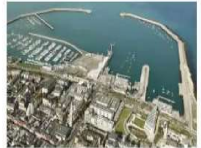
Coastal and harbor works
